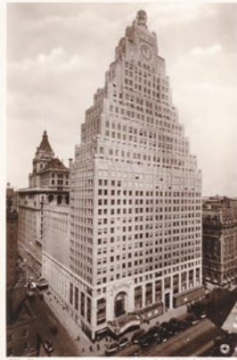
10781-78 PARAMOUNT THEATRE BUILDING, NEW YORK
